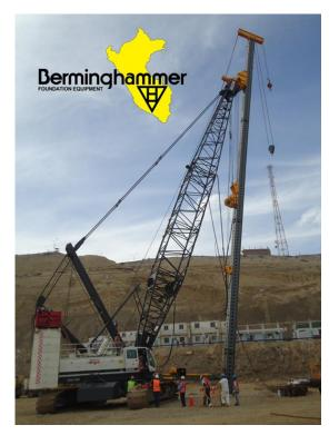
meters (134.4-ft) of L-27 Vertical Travel Lead system and a custom hydraulic retrofit kit for the customer's HC-275 crane. Mike Christensen and his team were invaluable as they built, in very short order, a hydraulic retrofit kit for the customer's crane and L-27 system.
